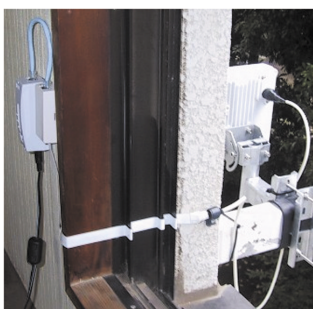
Fig. 6. Example of the installation of the window-frame-gap traversing unit.
