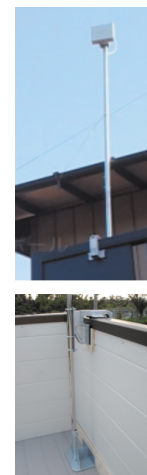
Fig. 10. Pole mounted on concrete fence.
