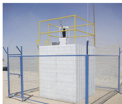
Fig. 4. Dust sensing facility. The roofed black cylinder is the measuring chamber of the dust sensor. The box below it houses a controller and a data collection device.
