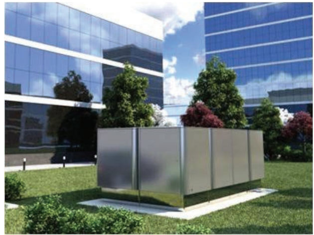
Fig. 5. 100-kw solid oxide fuel cell at a datacenter.
