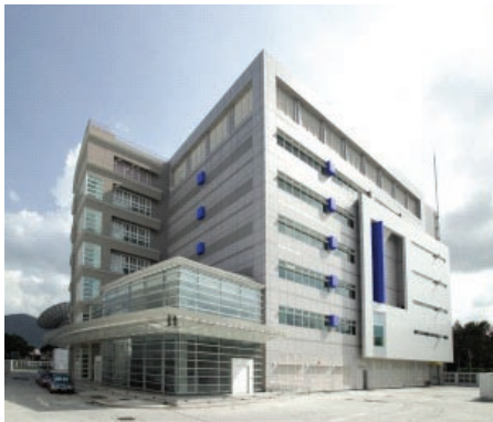
Fig. 1. NTT Communications Hong Kong Data Centre.
