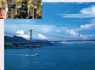
Tsing Ma Bridge.
