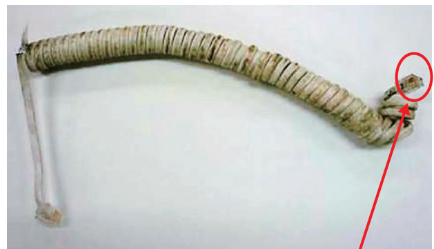
Broken modular plug
