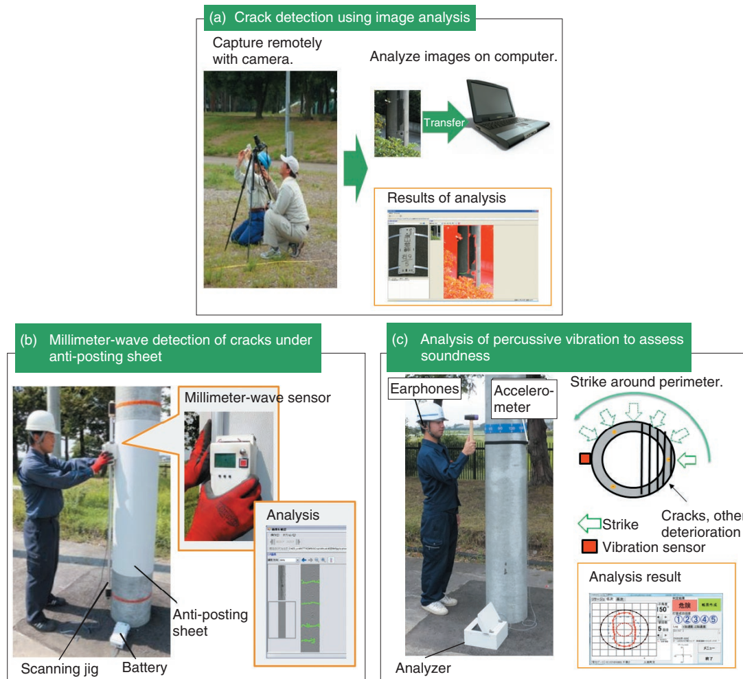
Fig. 4. Technology for inspecting concrete telephone poles.
