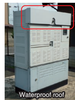
Fig. 8. Countermeasure to prevent penetration of rainwater.
