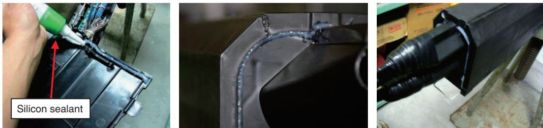
Fig. 6. Example of applying silicon sealant to a closure.
