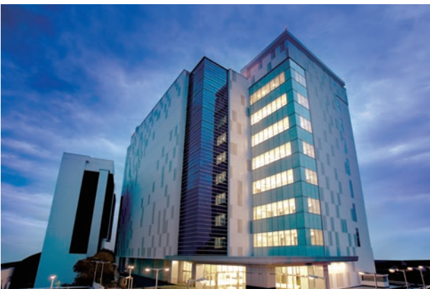
Photo 1. External view of datacenter in Jakarta.
