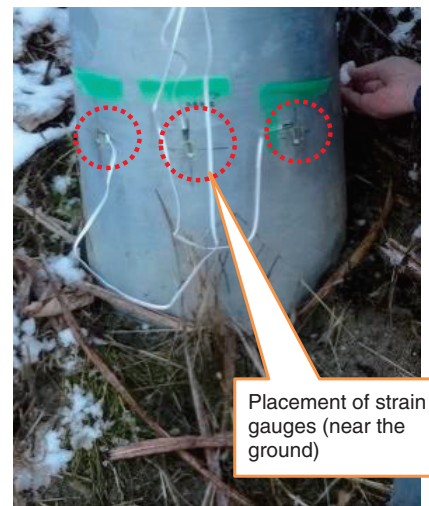
Fig. 4. Setup for evaluating applied stress due to snow pressure.
