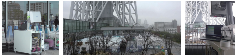
Construction of 5G communication environment at Sky Arena on 4th floor of Tokyo Skytree Town
