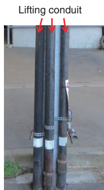
Fig. 2. Lifting conduits installed alongside a telephone pole.
