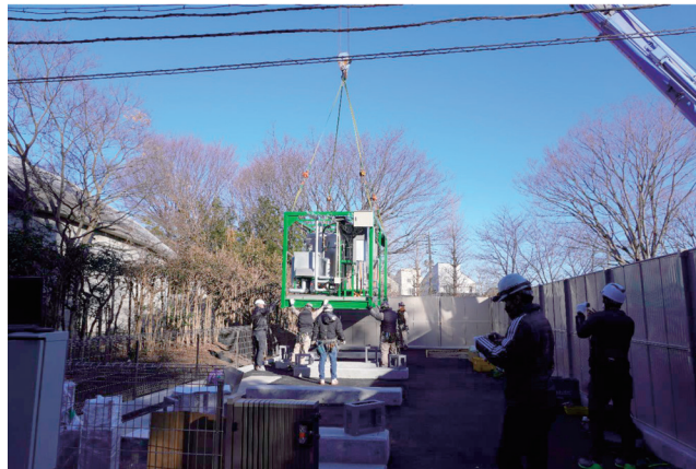
Fig. 2. Installation work for the container-type biogas plant.
