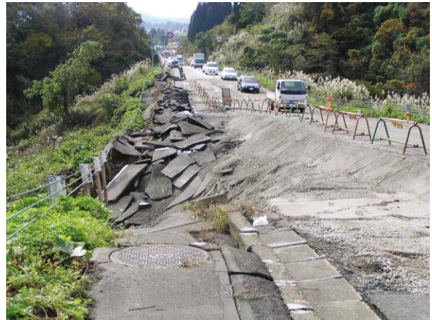
Fig. 2. Damaged manhole.
