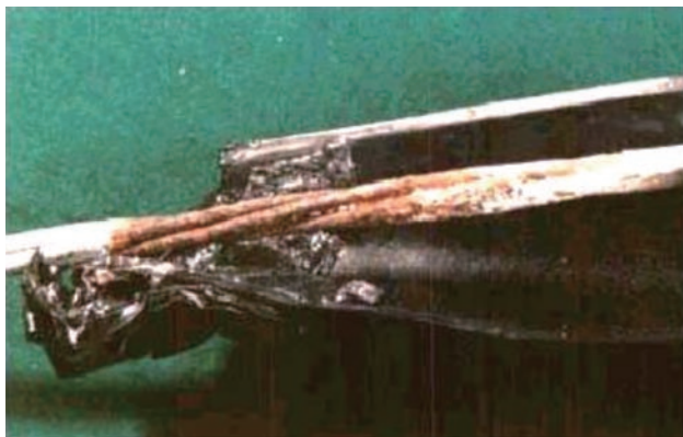
Fig. 3. Example of crevice corrosion in wire strand at connecting terminal assembly nozzle exposed to severe marine environment.
