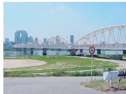
Fig. 10. NTT dedicated bridge (length: 800 m).
