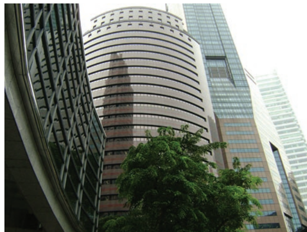
Fig. 2. Equity Plaza Building, in which the NTT Singapore office is located.
