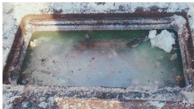
Fig. 1. Handhole prior to deicing.
