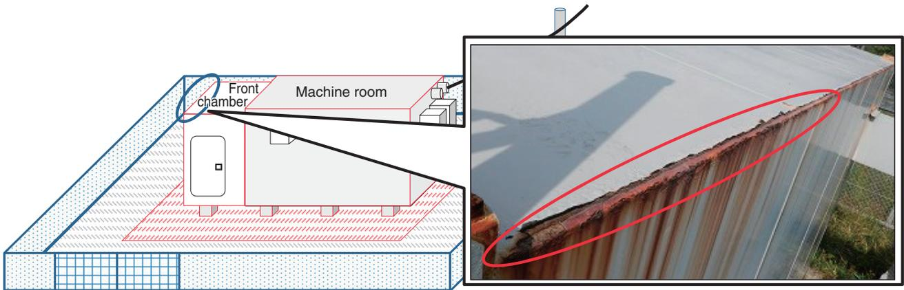
Fig. 2. Example of deterioration in RT-BOX steel.
