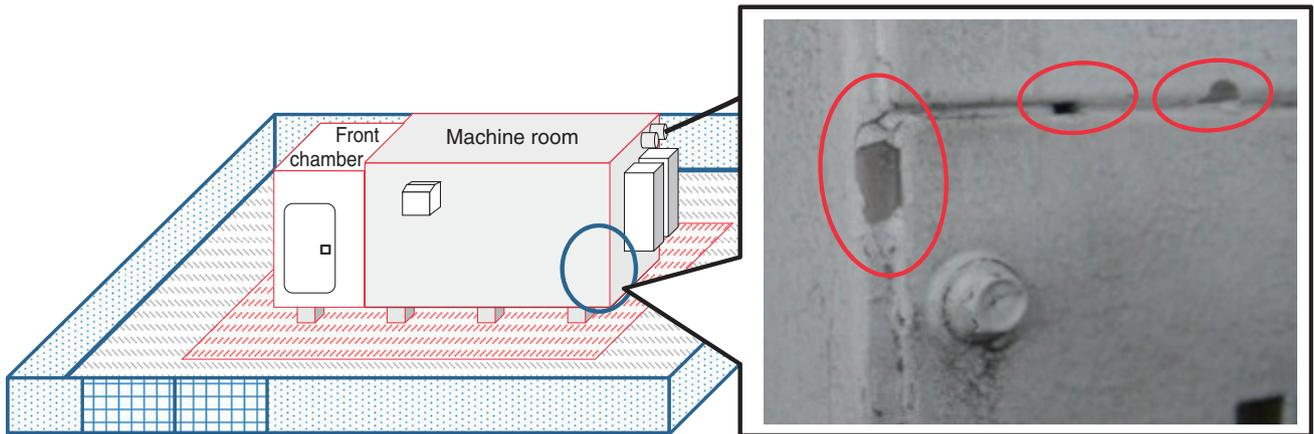
Fig. 3. Example of deterioration in RT-BOX paint.
