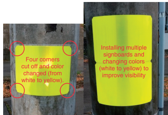
Fig. 9. Additional trial of signboard with adhesive backing.
