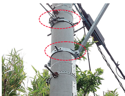
Fig. 5. Example countermeasure against sulfur damage to outdoor telecommunication facilities (metal bands with powder coating).
