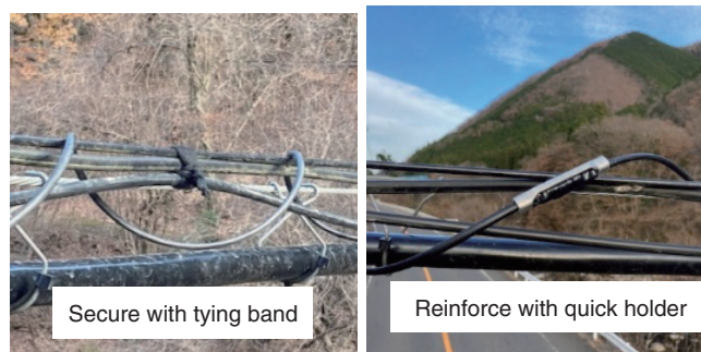
(a) Securing a cable
