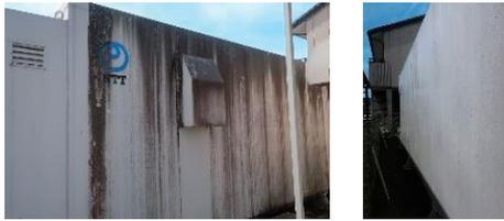
Fig. 2. Appearance of outdoor telecommunication box. Left: side with poor sunlight; right: side with good sunlight.
