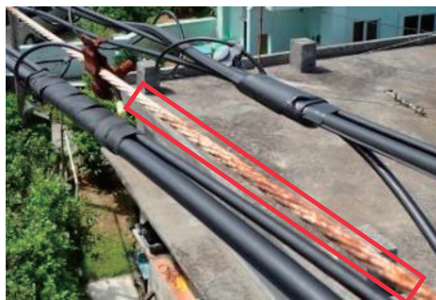
Fig. 1. Red corrosion on a messenger wire.
